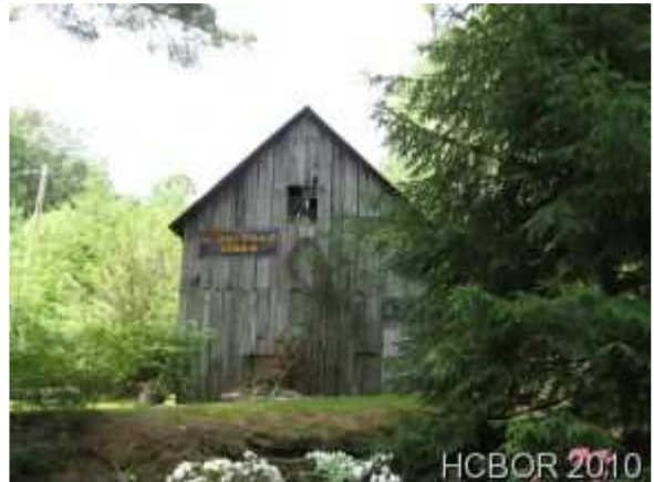
Old Barn Used For Storage
